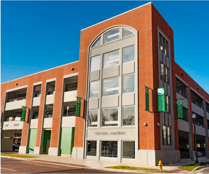
Four-level, 399-space, precast parking structure. This garage is located off the historic courthouse square in the City of Oxford, MS. This garage offers convenient parking for visitors and employees of local businesses, especially during Ole Miss fall football season and Double Decker Festival in the Spring.
